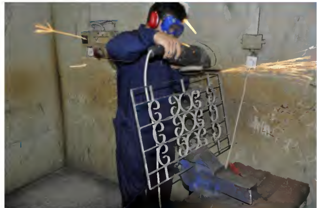
Ahmed is doing welding for maintenance works at NECC premises
